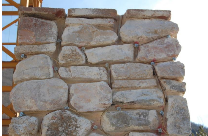
Figure 5. “Reticolatus”, an innovative technique for repointing of irregular masonry
