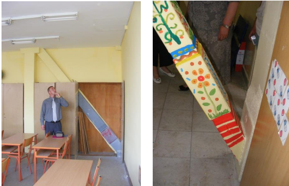
Figure 1. Vertical stiffening in longitudinal Y-direction diagonal square cross-section 260x160x7 with damper. Force in damper \pm 1100 kN, displacement \pm 5 mm.
