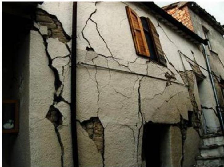
Figure 3. In this masonry building it is possible to see a flexural wall failure. There is a good roof-to-wall connection but the middle floor is not connected to the wall. In this case we can see how important is to achieve the connection between the roof and the existing masonry.
