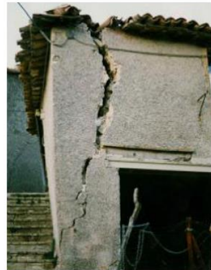
Figure 4. In this masonry building it is possible to see the overturning of the wall caused by a poor connection of the roof to the wall.
