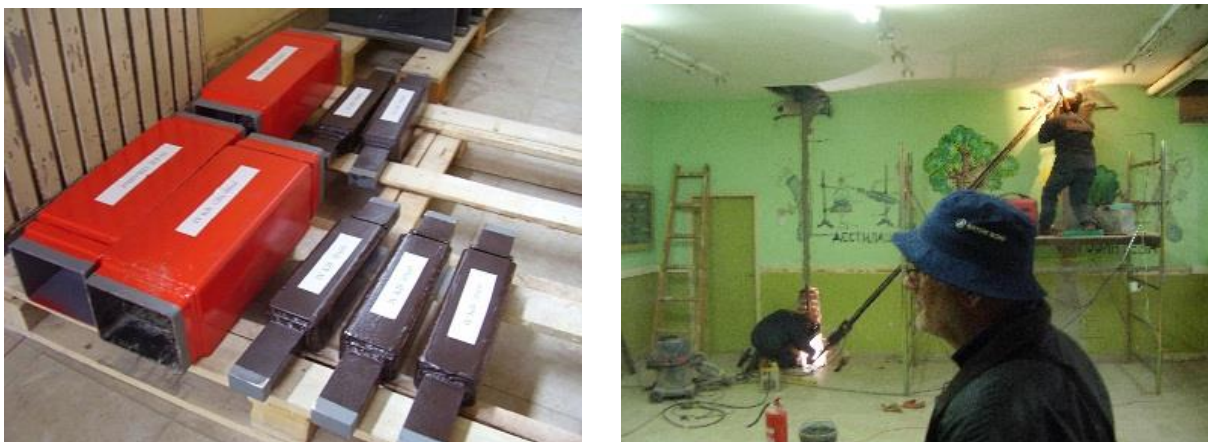
Figure 1. Part of Delivered Equipment-Dampers Figure 1. Connecting of verticals and diagonal with Damper by welding
