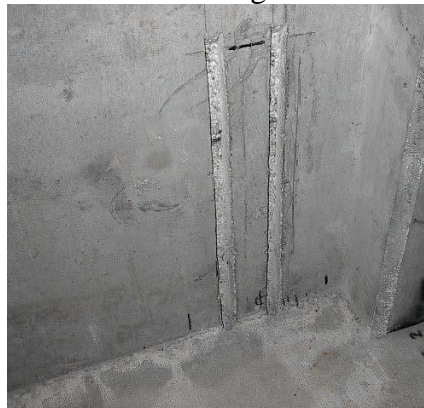
Figure 6. Reinforcement continuity at column/wall to footing connection: (a) FRP nail; (b) NSM FRP bar.
