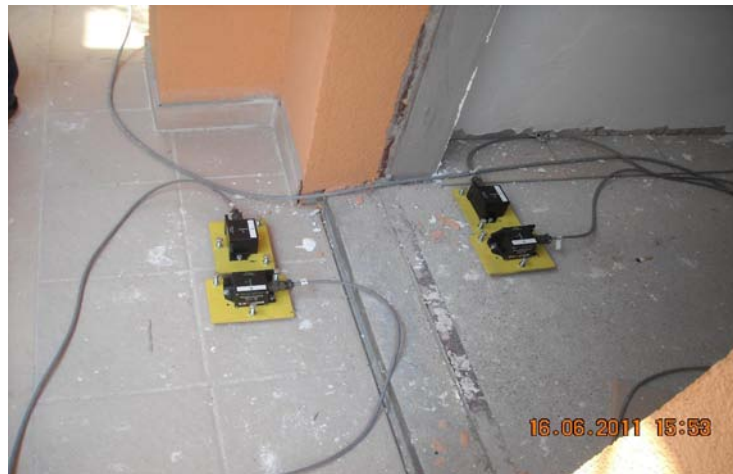
Figure 27 Separation joint- forced vibration test
