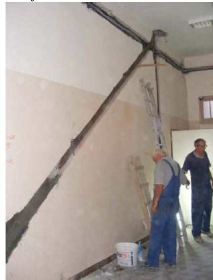
Vertical stiffening of the longitudinal wall in Agro-chemical school
