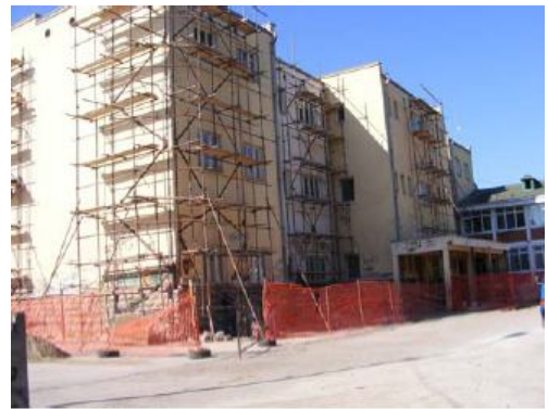
The Facade of the Primary school D. Tucovic
