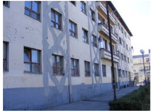
The Facade of the High school
