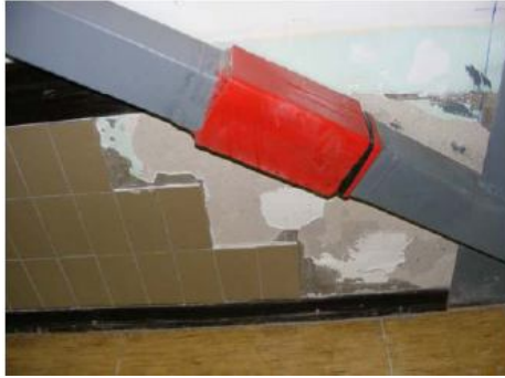
Absorber KN/5mm 1100 out wall plane in the High school
